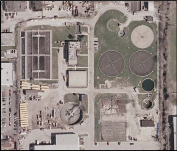
Bensenville Wastewater Treatment Plant.
